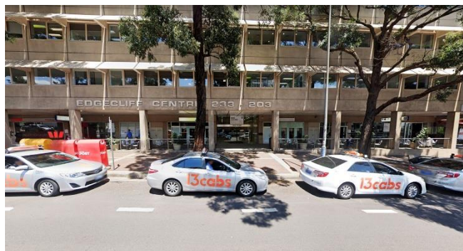
Figure 4 – Edgecliff Centre, viewed from the north
